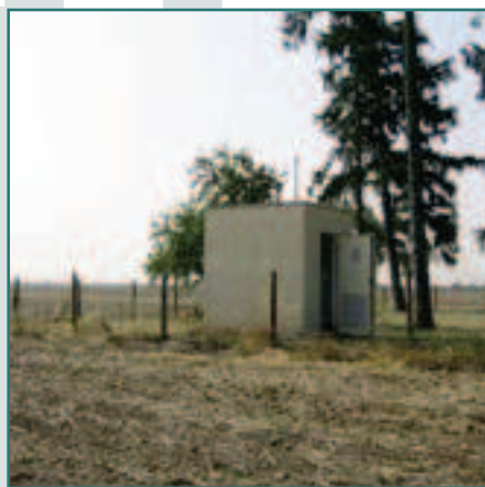
Station de surveillance de Oysonville.
