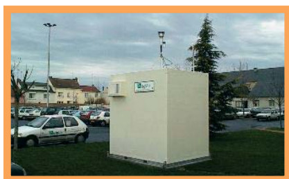
Station Châteauroux Sud
